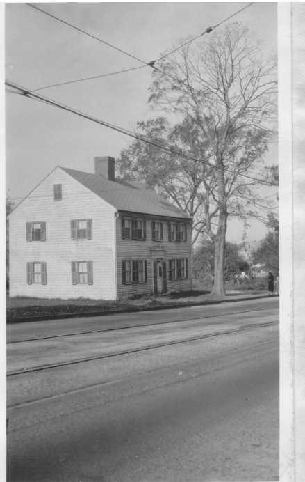
The Daniel Augur House Now owned by the Pease family (See page 37) Built about 1775 388 Main Street. No longer standing. Razed Now a gas station 1940 Oct. 1953
