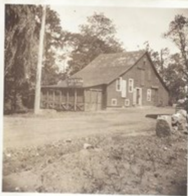
The site of the first ironworks in Connecticut built in 1688 Now owned by the Millerton Water Co. Farm Lane and Main St. (See page 3)
