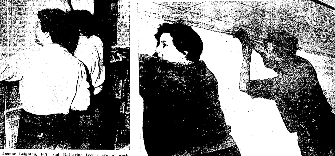
Marjorie Brown works with William Hasse to put up a strip of molding along the ceiling of the 'Drop-in Room'.
