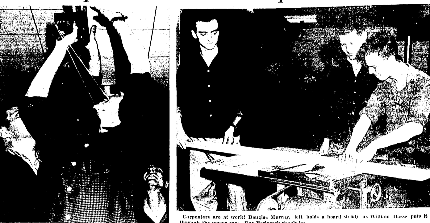
Carpenters are at work! Douglas, Murray, left, holds a board steady as William Hasse puts it through the power saw.
