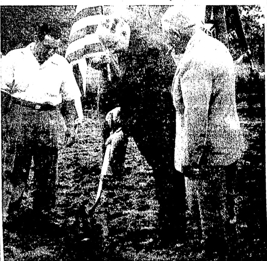
The Rev. Joseph Buckley, chaplain of the Father Regan Council, Knights of Columbus, turns over the first shovel of earth at the Roma Street site of the new $10,000 Columbus Club, while Grand Knight John Tinnari (right) and James Canna (left), chairman of the building committee look on.
