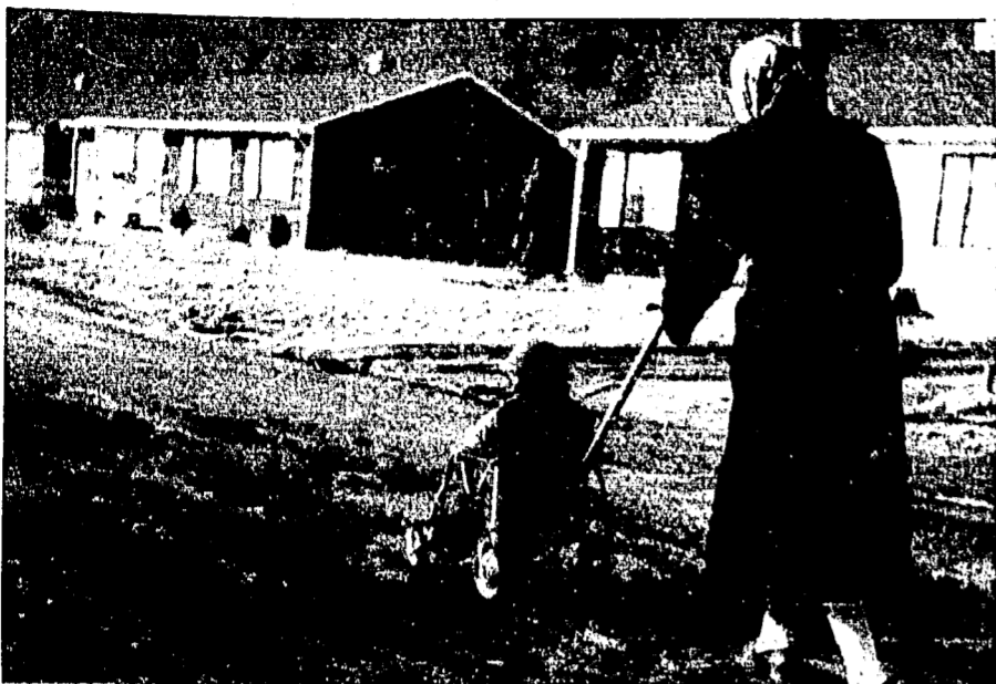
A protest movement over the condition of roads in High Ridge continued this week although repair work has been started by the sub-contractor in charge. Above picture was taken several weeks ago on Van Horn Dr.
