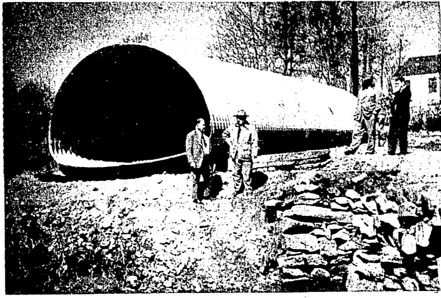
Shown above is a giant corrugated steel culvert which is being readied for placement as part of a bridge over a creek crossing under Mansfield Rd. The culvert, assembled under state supervision, is a new type of waterpass. Town and state officials are shown inspecting the dredged out creek-bed into which the culvert will be dropped by crane.
