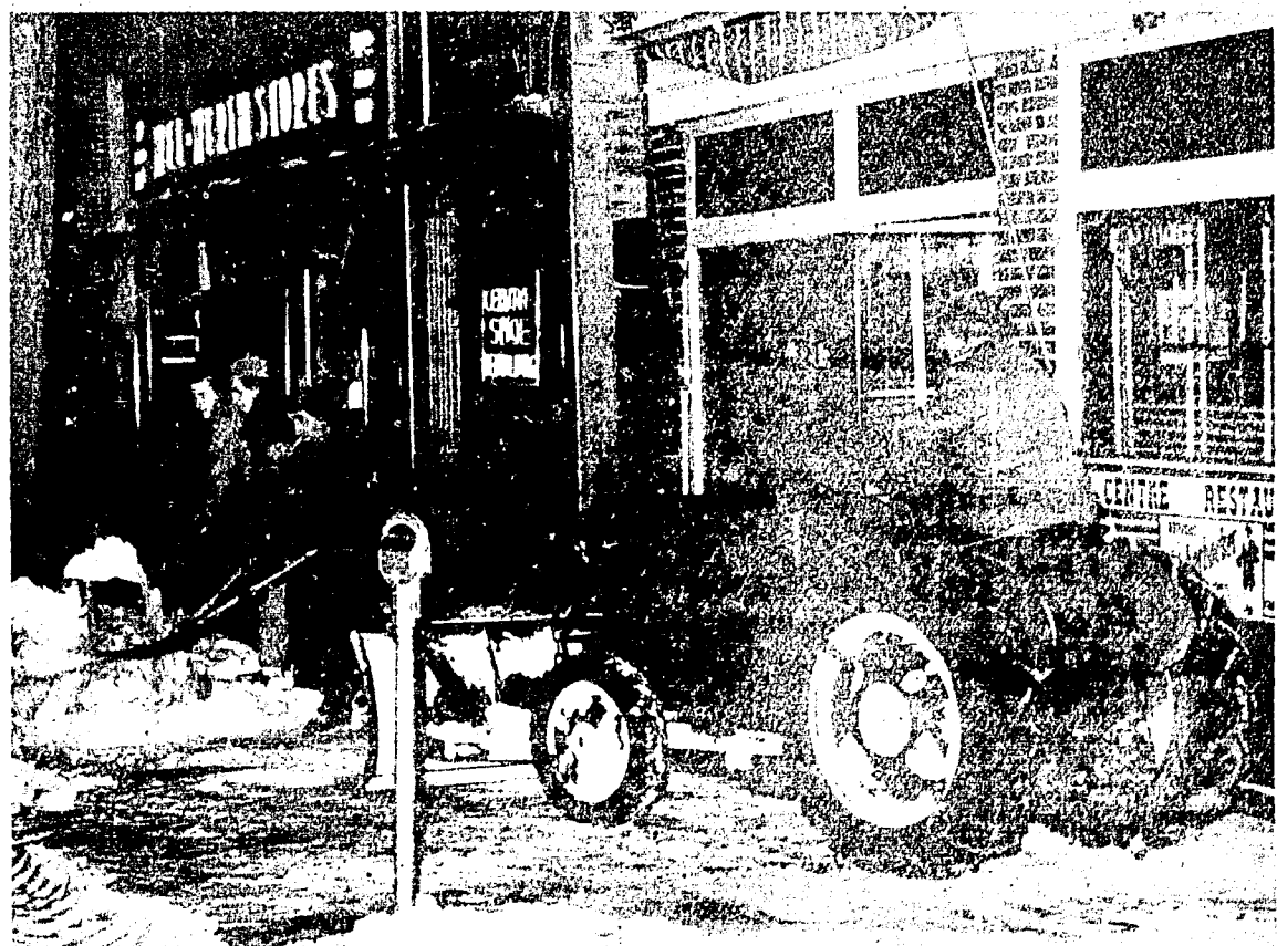
Members of Town crews join with a rented plow to clear the sidewalks on Main St. of the heavy snow fall. Crews worked the clock around, to clear the way for both autos and pedestrians. This picture was taken at 3 a. m. Tuesday morning. Operating the plow is John Limonecchi, local contractor, and brother of Peter Limonecchi, of the Board of Public Safety.
