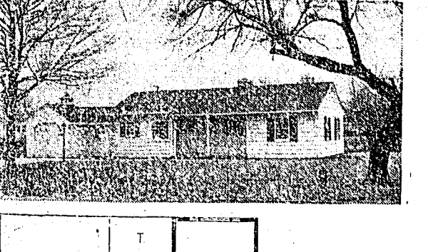
Containing six rooms with an attached garage, this house is well adapted to a corner lot site...
