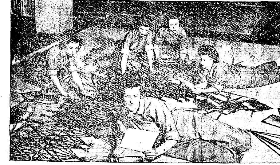
These WAVES are working on a jig-saw puzzle—the most important jig-saw puzzles imaginable. On duty at the Navy Hydrographic Office, they are helping construct a chart by use of aerial photographs. In its form the chart will guide the Navy's fighting men in operations in the Pacific zone. In existence two years, there's still need in the WAVES for thousands of patriotic young women—20 to 35, without children under 18—whose starting pay, counting food and quarters, will be $14.50 a month, plus many "extras" and post-war advantages.
