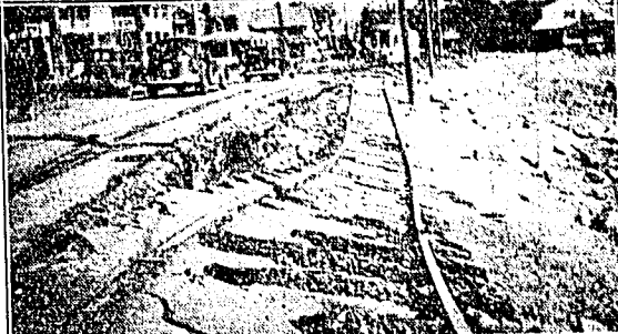
A section of the retaining wall washed out at Short Beach in the recent hurricane. The Town meeting last night voted 103-47 against the motion to erect another. Picture taken by Mrs. A. J. Pfeiff of Short Beach a week after the storm.
