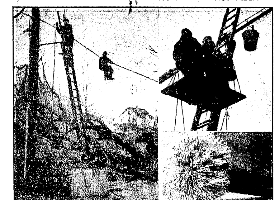
The unique crafts of the cable splicer—whose work plays such an important part in restoring hurricane-wrecked telephone service in Connecticut—is graphically shown in these pictures. At the left, after new poles have been erected, a strong steel wire is suspended on them, and a man "rides the line" placing rings at regular intervals. Then the new cable is piled through the rings. At the right, above, is shown a splicing crew at work; each individual wire must be identified in both the cables that are being joined, then they must be twisted together, properly insulated from each other, and finally all the wires are covered with a lead sleeve and sealed with solder to make the splice waterproof.
