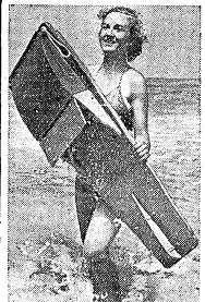
Miss Althea Martin shown with the new type of surf sled patented by a Los Angeles newspaper man, which will lessen the danger of the rider getting hurt in the surf. The streamlined pontoon below its nose allows it to float the rider in perfect safety, while the stabilizer shield along the tail holds it to a straight
