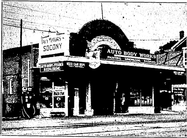
Above, is a photograph of the old Talmadge Garage, which has recently been taken over by Tacy Motors, Inc., as their auto body works, directly across the street from them. To the right may be seen the Old Bridge Package Store; one of the nicest stores of its kind in East Haven.
