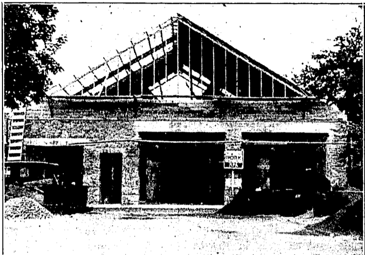
Above, is seen the Town Shed under construction, which is being built in the rear of the Fire Dept., Co. 1, in Main Street. If you look closely you can see the old shed in the center.
